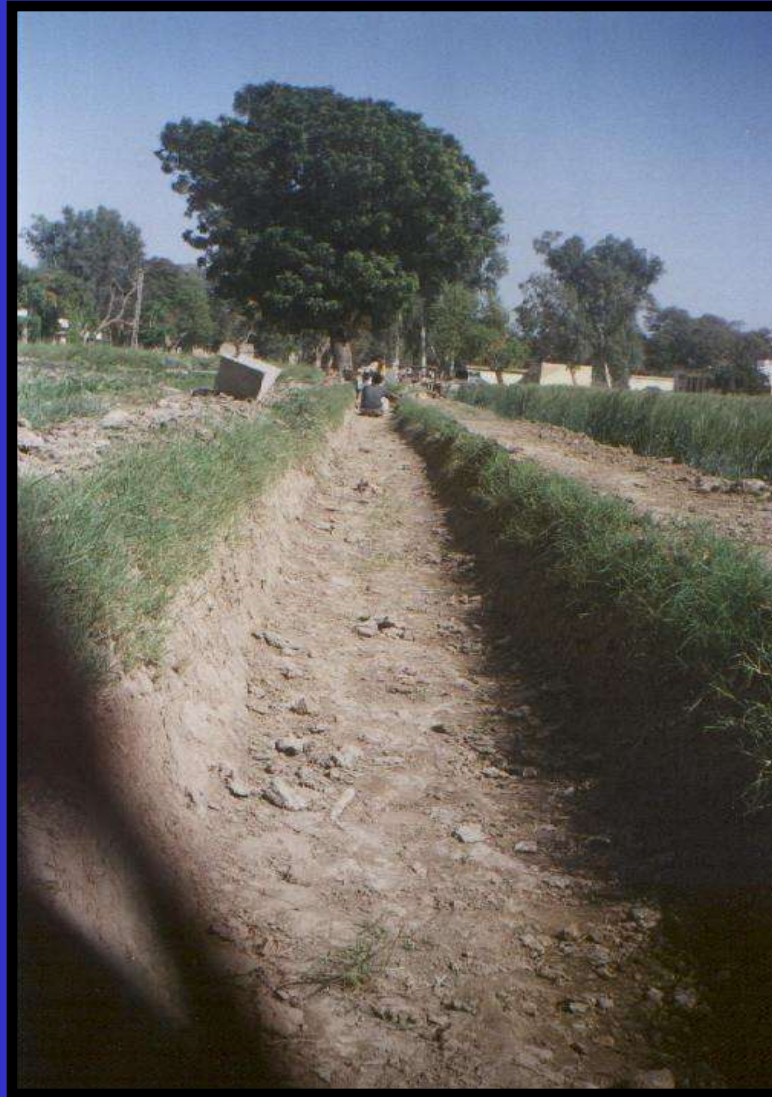
View of unlined channel at Tandojam
