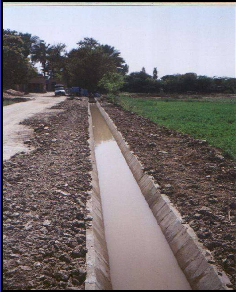
View of channel lined at Mirpurkhas with Precast Lining Unit Developed by CWHR.
