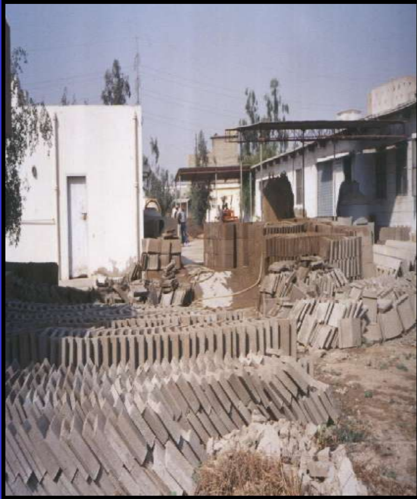
Stock of precast lining units at CWHR
