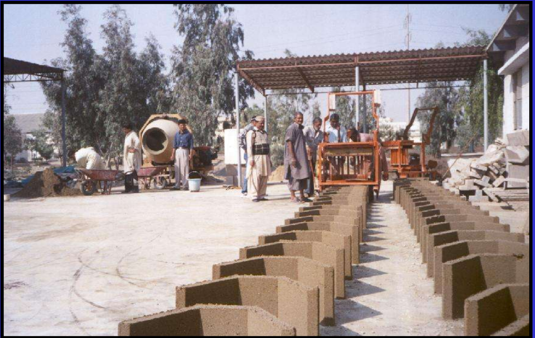
Casting of Precast Lining Units at CWHR yard
