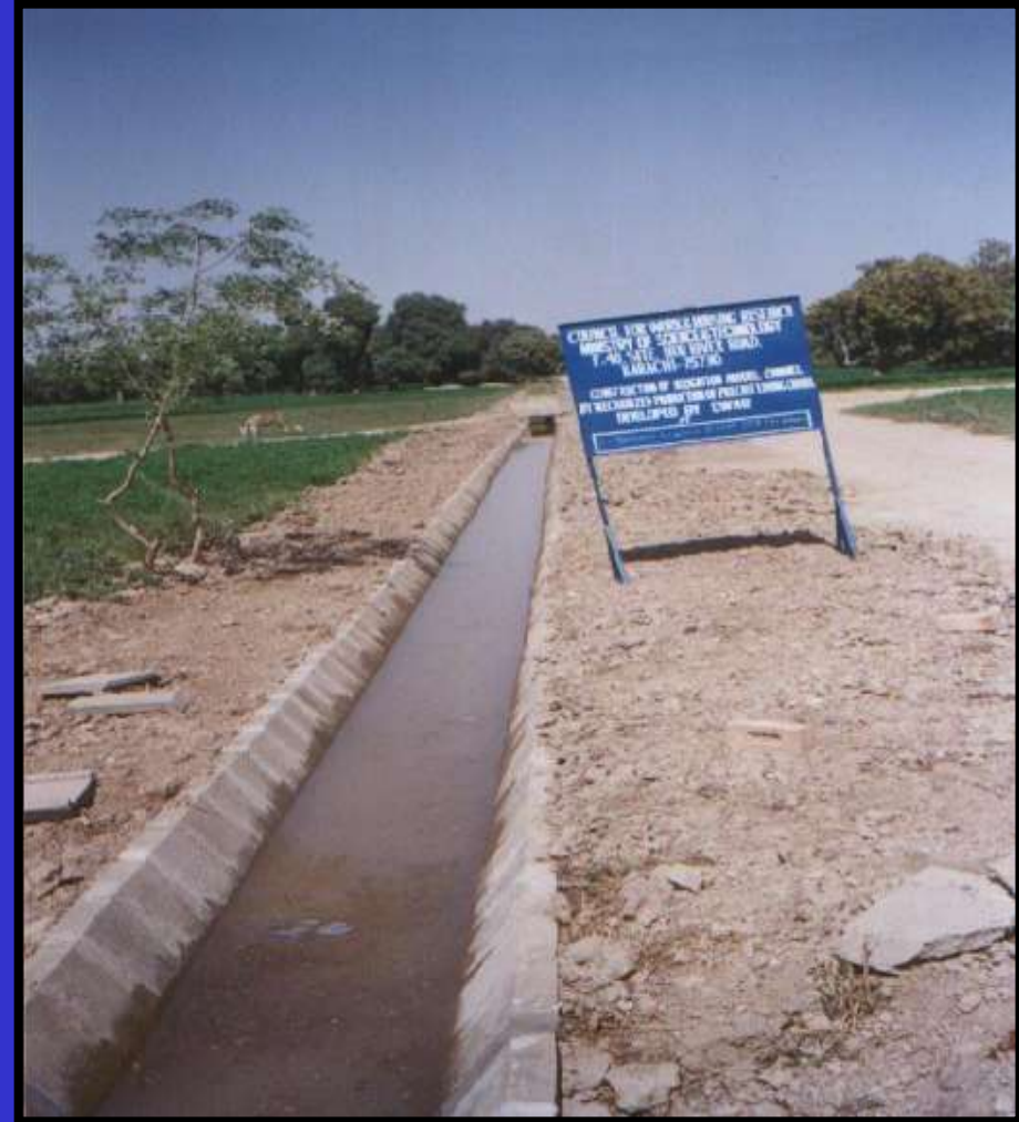
View of channel lined at Mirpurkhas with Precast Lining Unit Developed by CWHR.
